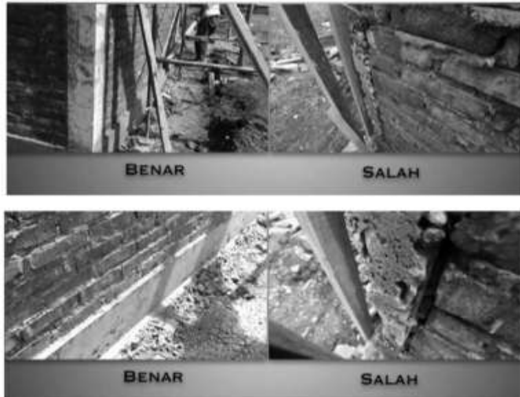
Gambar II.417 Hasil Pengecoran
