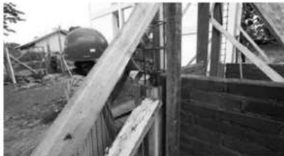
Gambar II.415 Proses Pengecoran Kolom
