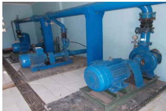
Gambar 3.4 Pompa Distribusi IPA Pinus
