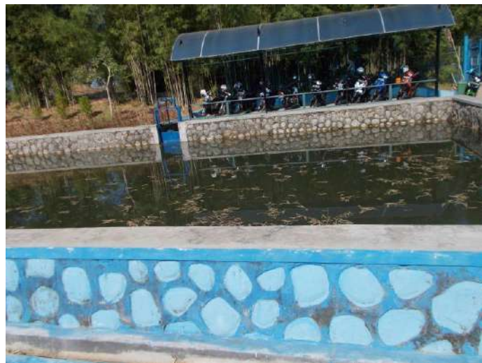
Gambar 3.11 Unit Prasedimentasi PDAM Intan Banjar
