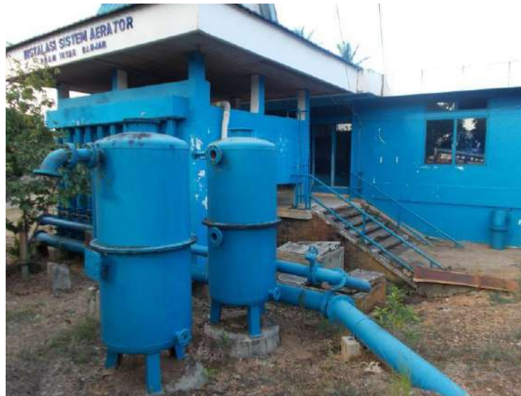
Gambar 3.28 Pipa Distribusi (transmisi) IPA I STM (Aerator)
