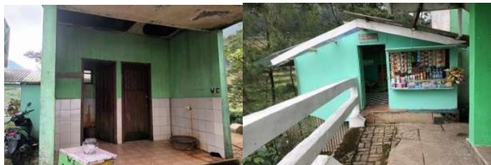
(a) Fasilitas Toilet
