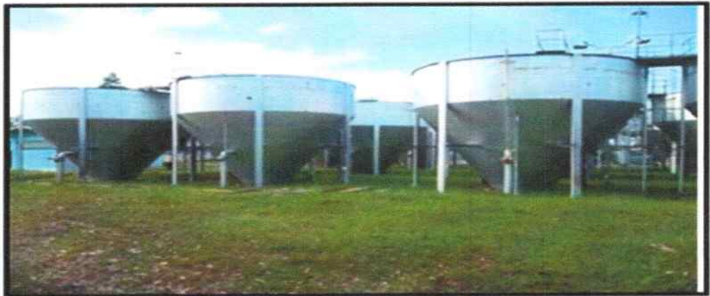
Gambar 3.15 Accelerator
